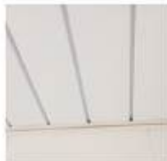
Interior ceiling tiles
